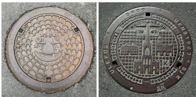
Fig 1. Two Norwegian examples of manholes designed to be opened with a specialist lever tool
